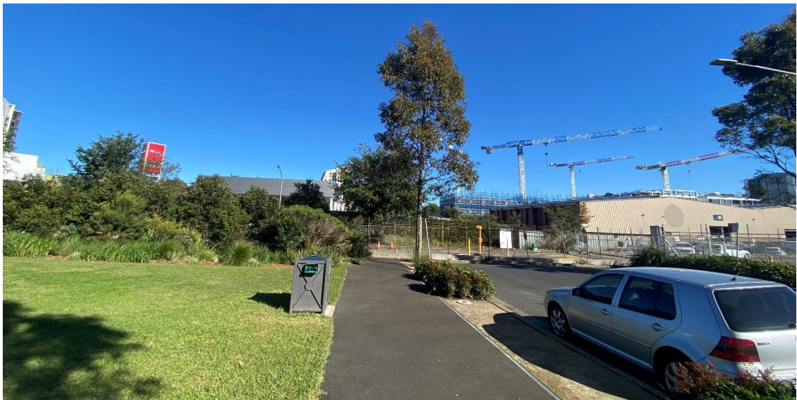
Figure 7 Subject site as viewed from Defries Avenue
